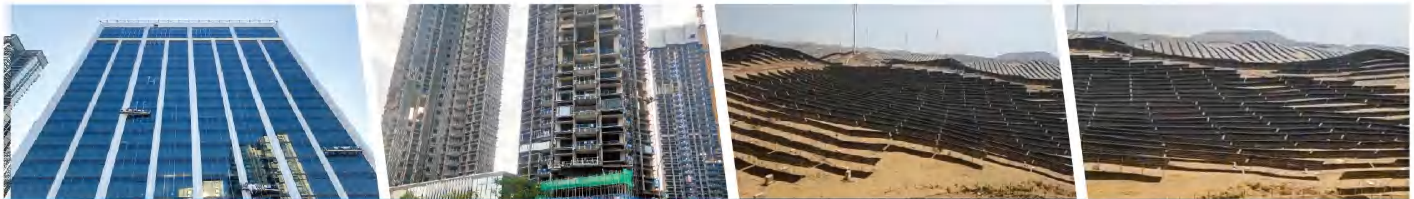
▶ Huawei Antoine Headquarters Building Project
