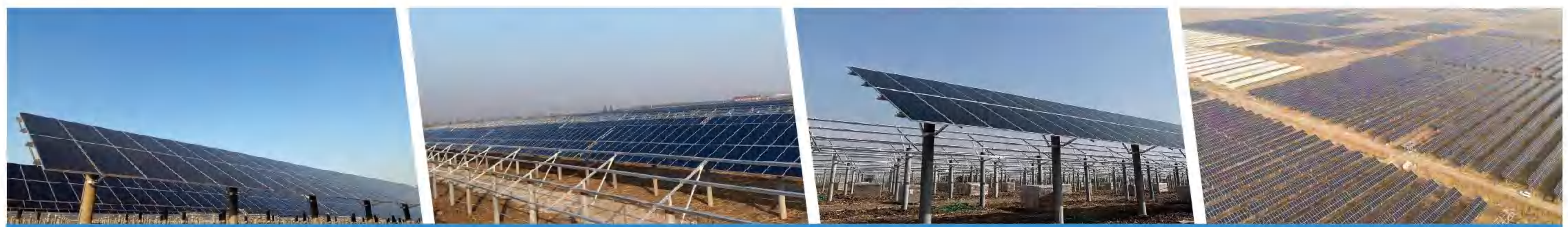
▶ Heilongjiang 200MWp Ground Station Project
